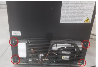
• On the back of the unit, remove the 4 Phillips screws securing the grated cover over the back of the
