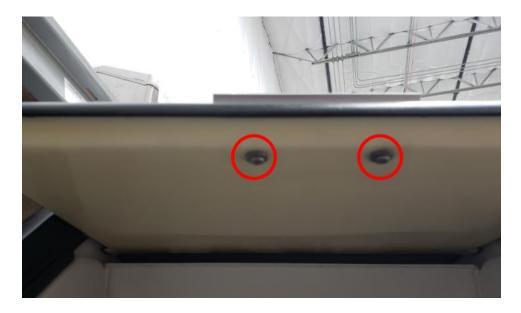
Step 7: Reinstall the top panel of the unit
