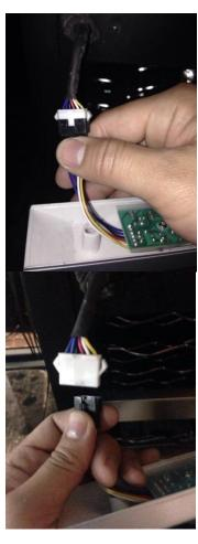
5. Reconnect the wire connector and reassemble the control panel.
